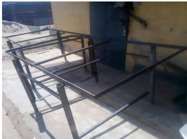
Figure 3: Assembly of metal structures
