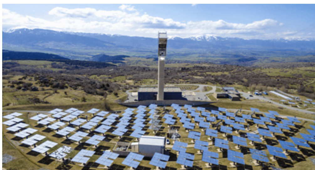
Figure 1. The Thémis solar plant of PROMES-CNRS in Targassonne (France). For one heliostat in the solar field, canting errors were quantified and rectified with terrestrial laser scanning, and the resulting change and improvement in the solar flux distribution at the flux target below the receiver was assessed.
