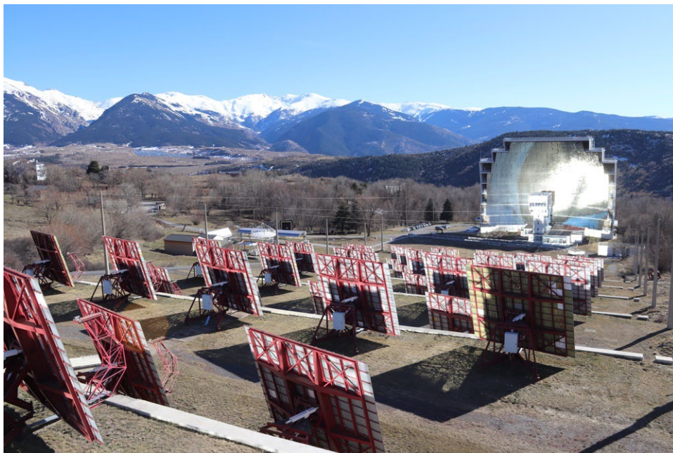
Figure 1. Overall view of the Big Solar Furnace and heliostats in Font Romeu Odeillo, Eastern Pyrénées, France, operated by the PROMES-CNRS laboratory since 1968.
