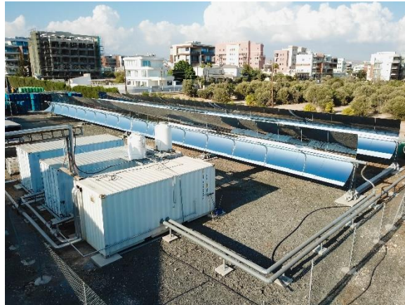
Figure 1. View of the PTC system and C-TES at KEAN Soft Drinks Ltd (Photograph © Protarget AG).
