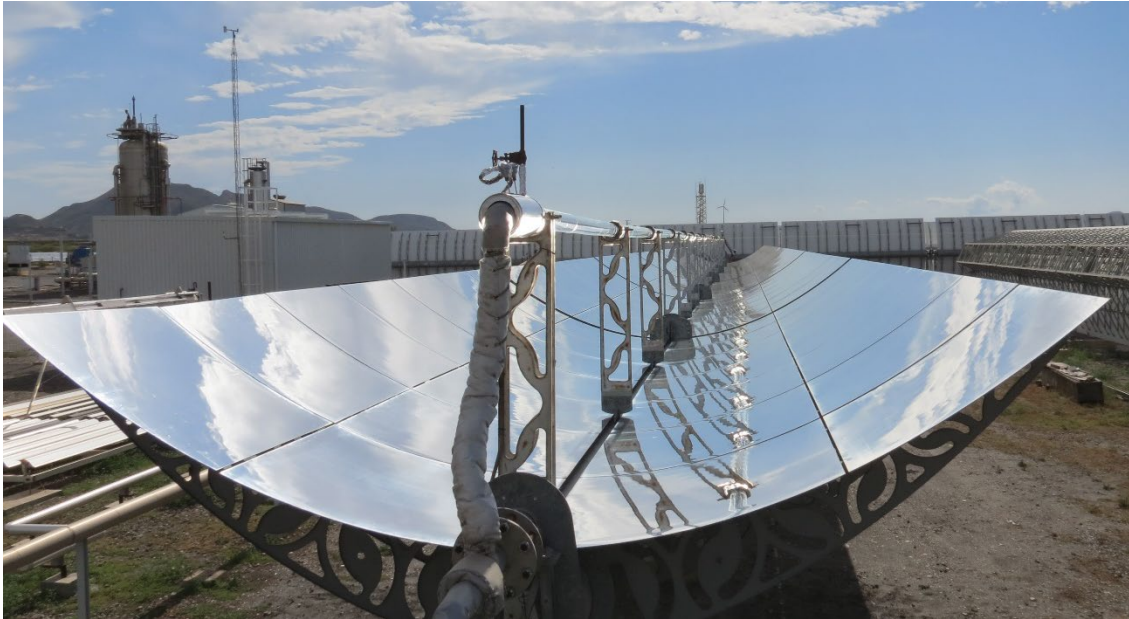
Figure 2. View from the west of the UrssaTrough parabolic trough at the Plataforma Solar de Almería (east-west orientation), with a ROTAJOINT connector installed at the collector outlet. (Note: Fluid flow direction to the camera).
