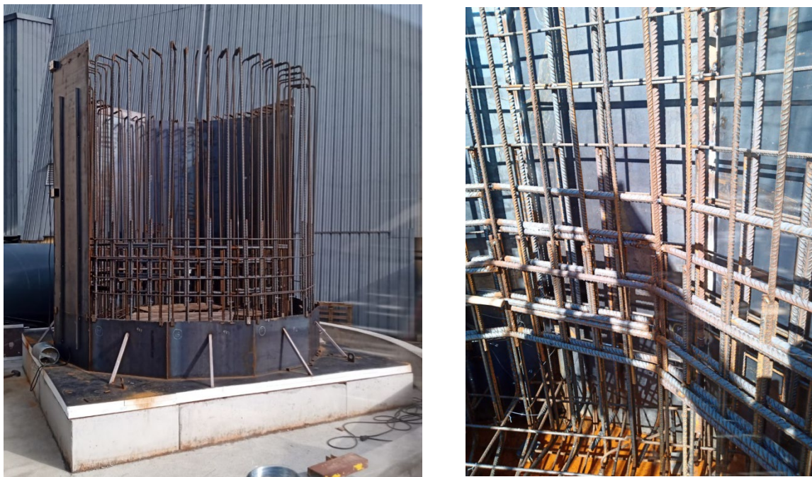
Figure 4. Reinforcement view while erected and detail from inside.
