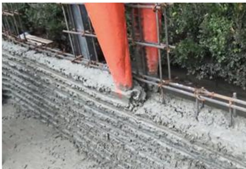
Figure 1. Simultaneous extrusion on both sides of the steel reinforcement cage [9].
