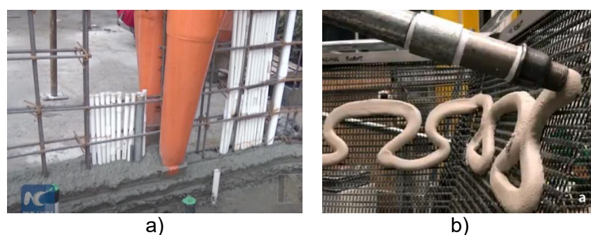
Figure 1. Introduction of reinforcement prior concrete printing: a) 3D printing around the steel meshes using bifurcated printhead [17] and b) extrusion-based material deposition on a fine textile mesh [18].
