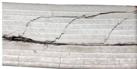
Figure 9. Ultimate shear failure in the thickness of the beam, initiated under the load.
