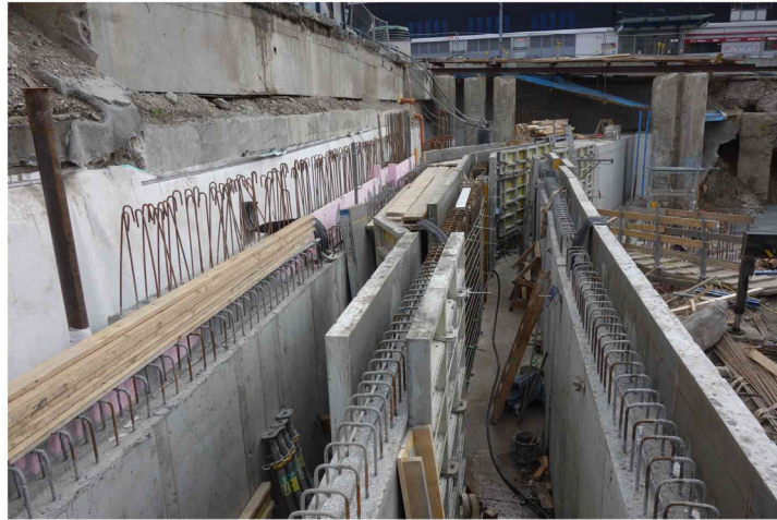
Figure 2: Construction of two parallel sewer lines (Wiedemann, Rabmer GreenTech GmbH).
