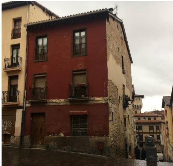
(a) Pre - Renovation
