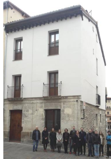
(b) Post - Renovation
