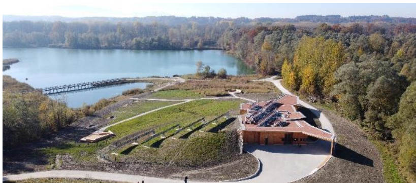
Figure 1. Aerial view of the building Auenwerkstatt, source: RES Renewable energy Systems GmbH.
