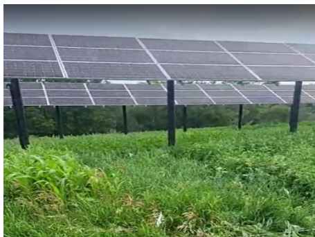
Figure 1. Forages underneath the 30kW solar ground-mounted array site at the University of Minnesota West Central Research and Outreach Center in Morris, Minnesota, USA.
