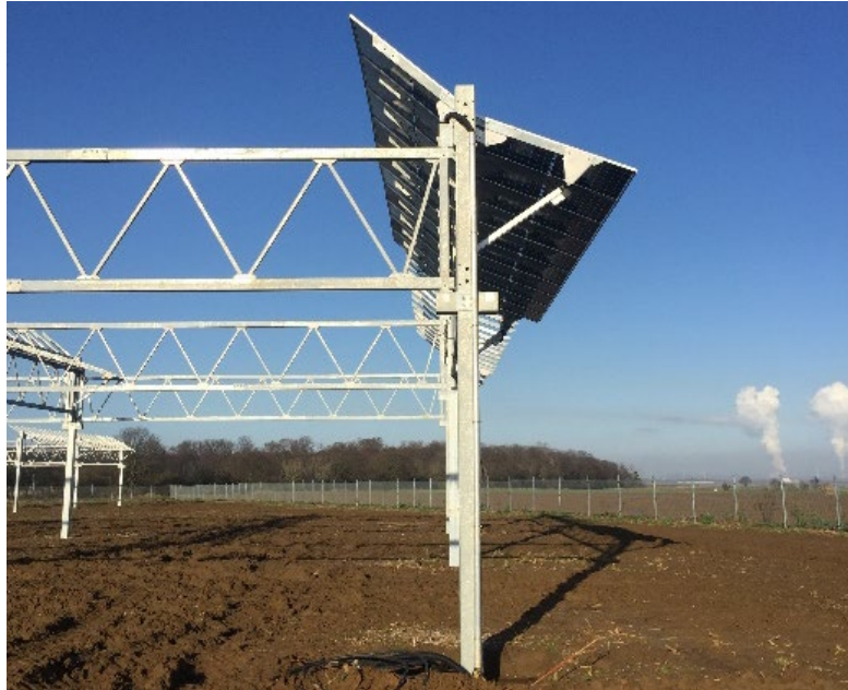
Figure 3. Side view of module V-shaped row with internal angle for rainwater harvesting capabilities. During rain events, the modules change to a zenith orientation for collection.
