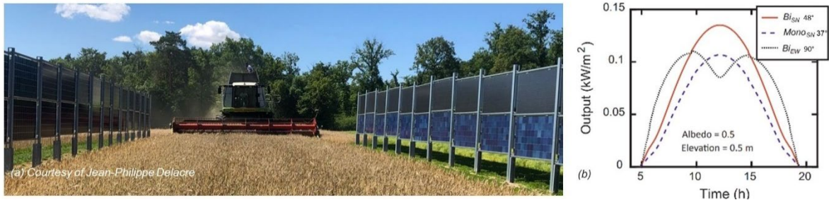
Figure 1. Illustration of (a) the vertical PV compatibility with crop operations (agrivoltaic system of TotalEnergies at Channay) and (b) the typical bi-modal production of east-west oriented vertical panels [3].
