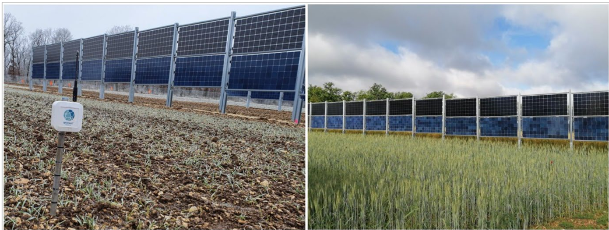
Figure 8. Agrivoltaic system of TotalEnergies at Channay in central France (left picture shows tensiometers that are used and right picture shows wheat growing in the system).
