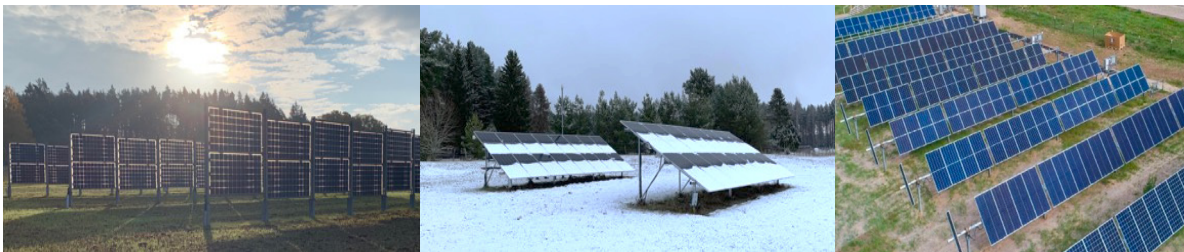
Figure 1. Photographs of the vertical AV system (left), GM fixed-tilt system (middle) near Västerås, Sweden and the 1-axis tracking system (right) in Golden, USA [5].
