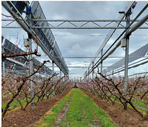
**Figure 1.** View of the 'Kinolea' nectarine orchard during bloom. Contrary to the picture, panels were in horizontal position during the night with frosts.
